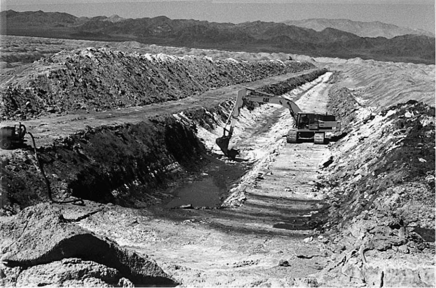
Figure 2.49 Backhoe cleaning salt from a seepage trench at Bristol Lake. (Courtesy of National Chloride Company of America).
