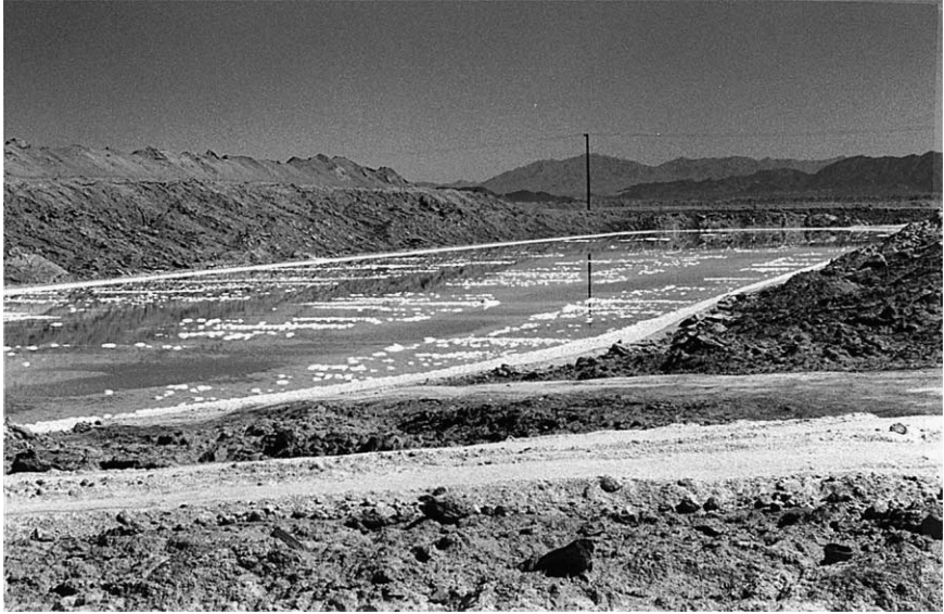
Figure 2.51 A typical brine holding (evaporation) pond at Bristol Lake. (Courtesy of National Chloride Company of America).
